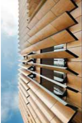
VERTICAL TIMBER LOUVRES
